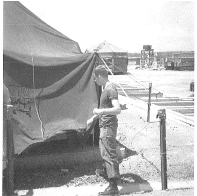
Sgt. Glenn Martin preparing to tie down a tent after erecting the frame 1966.
