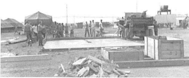
Enlisted personnel laying foundation for first Adam's pre-fab building 1966.
