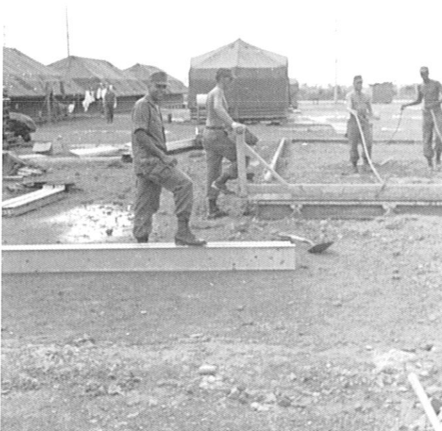
Major Beck, Detachment Commander supervising building of Adam's hut building 1966.
